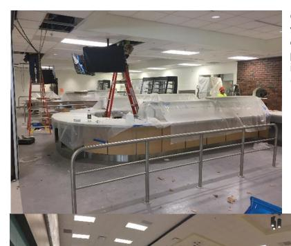
**CAFETERIA/KITCHEN** – Working on brick veneer at pizza oven, and above ceiling IT connections in Serving Lines. (top left photo). completing metal wall panels installation, and staging FF&E in Cafeteria. (bottom photo).
